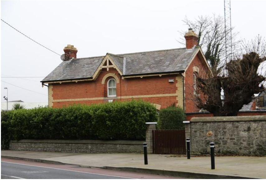
Plate 9.10: Former station master's house
