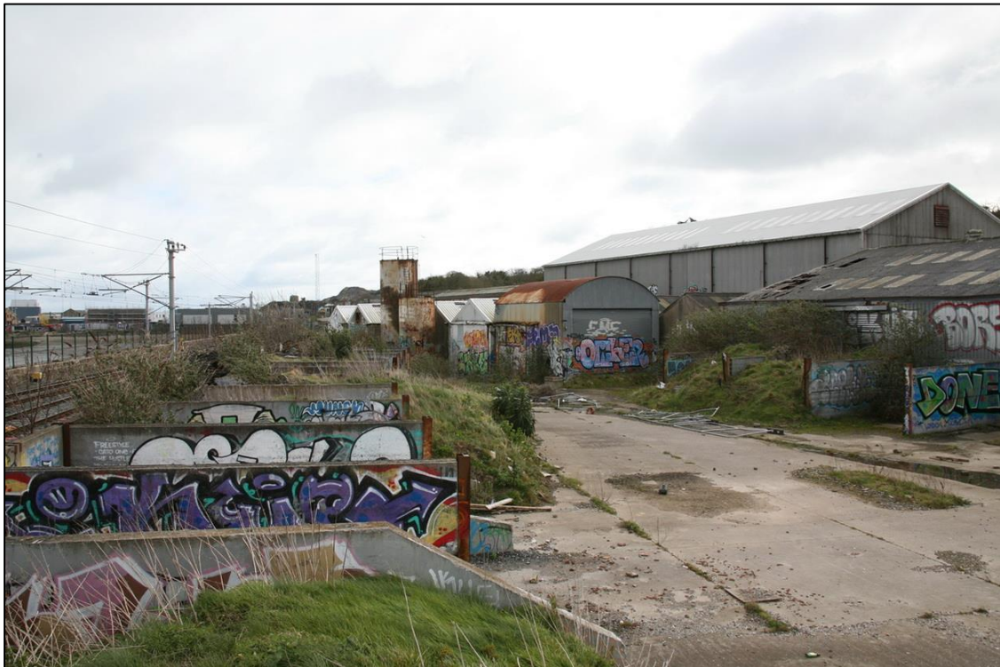
Plate 9.4 Techrete structures, looking southeast
