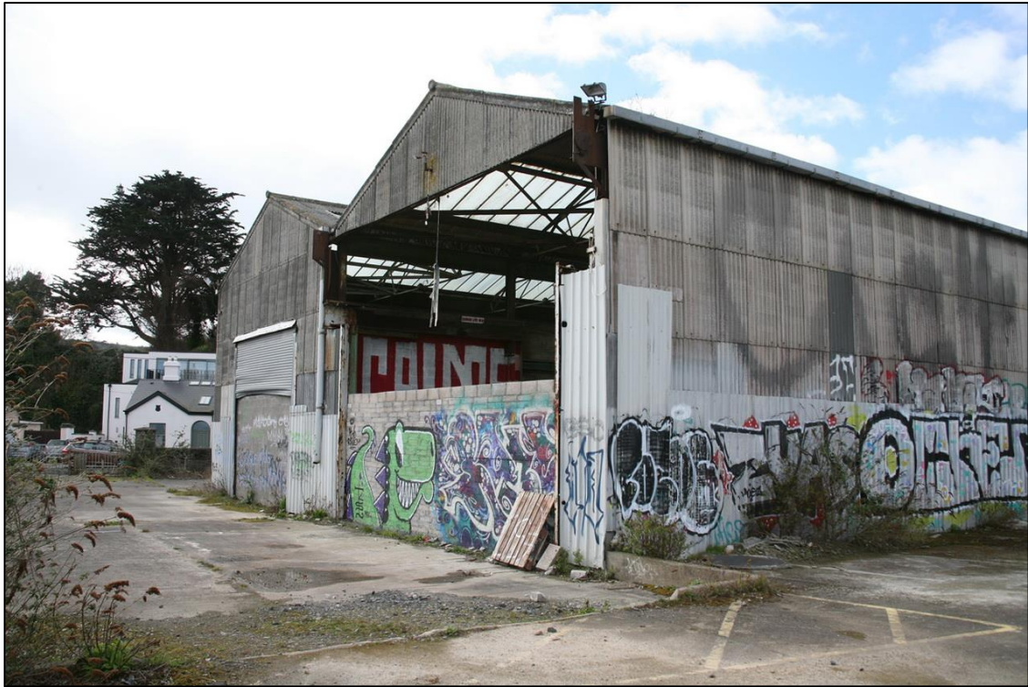
Plate 9.5 Eastern end of Techrete structures, looking south
