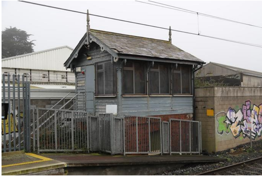
Plate 9.12: Signal box at Howth Railway Station
