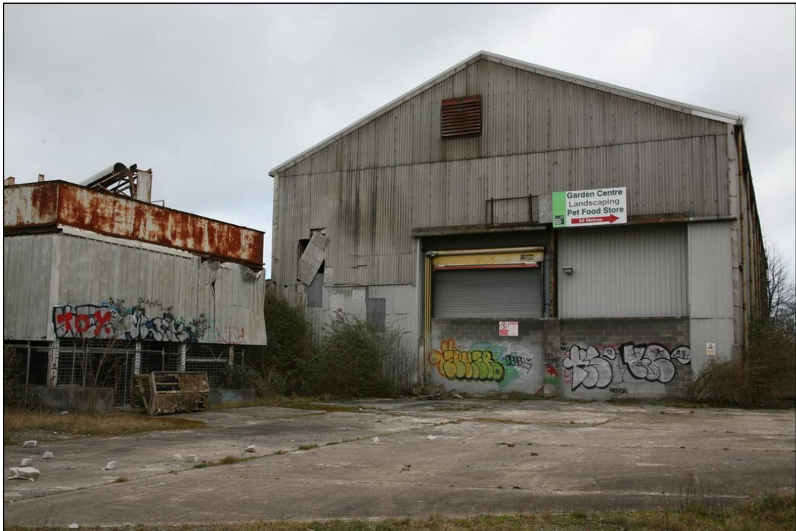
Plate 9.6 Western end of Techrete structures, looking east
