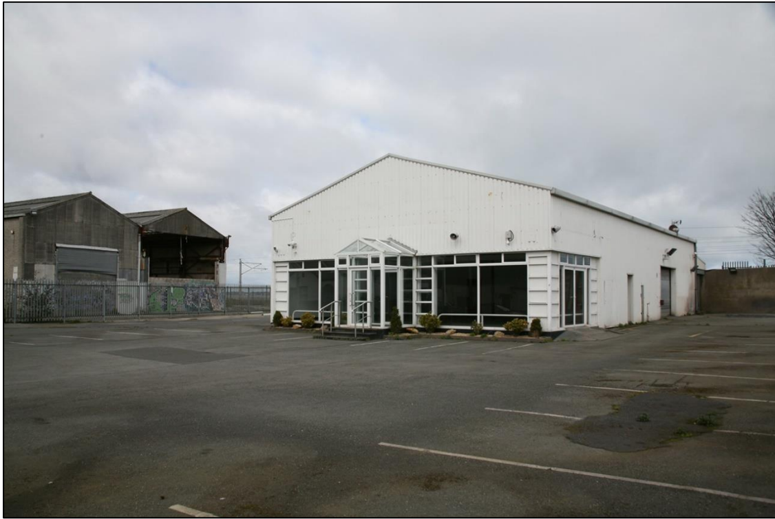
Plate 9.7 Former Beshoff Motors premises at eastern end of proposed development site, looking northwest
